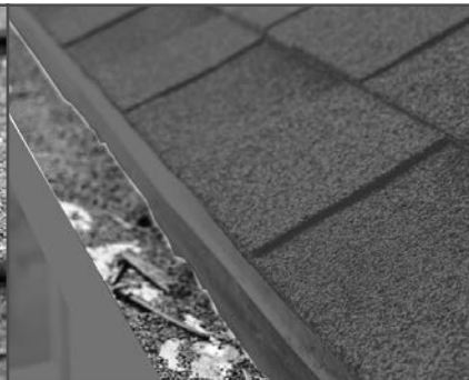
Granules in the gutter indicate shingle deterioration.
