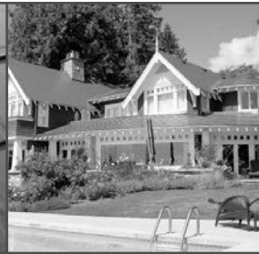
Metal roofing manufactured to resemble asphalt shingles offers metal's durability but blends with the look of other houses on the street.
