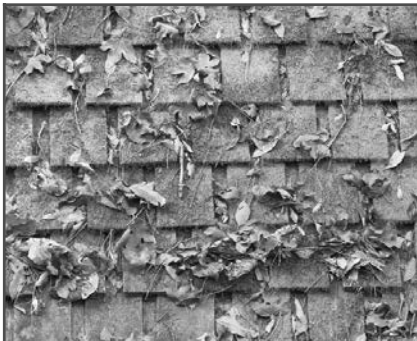
Shingles stained by algae are unsightly and retain moisture that can lead to premature failure.
