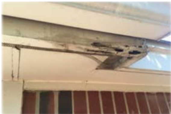
Here there is rot on the trim surrounding the soffit and fascia. This will increase the cost of your project for the cost to repair and replace the rotted boards.
